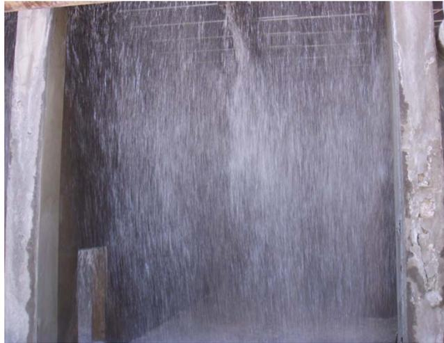
Figure 2b | Warm water spray inside the central plant cooling tower
